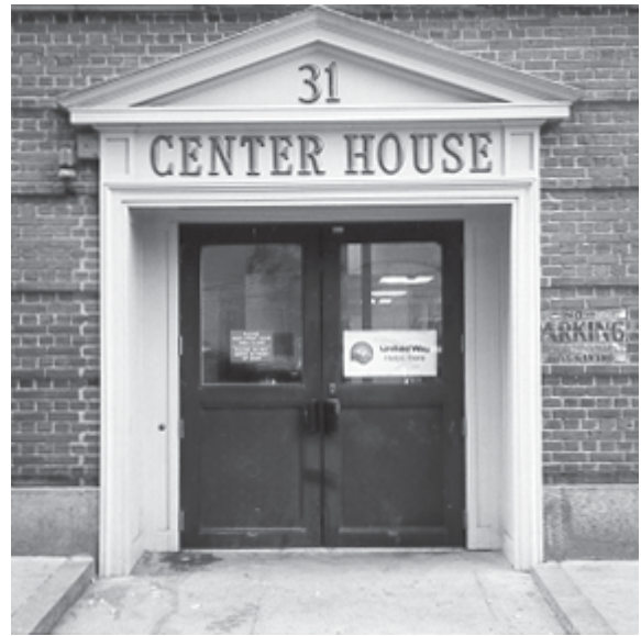
The Center House Day Treatment Program is located on the fourth floor of a five story brick building.
