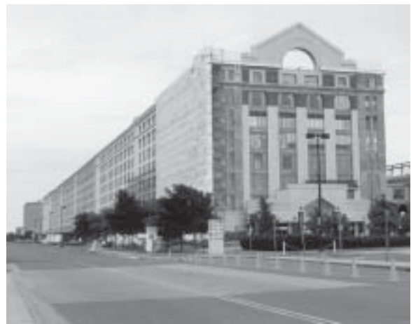
The Education & Training Program is based in a large building featuring commercial and light manufacturing activities.
