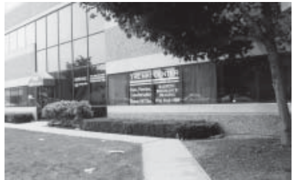
ASAP outpatient services are located on the second floor of a two-story office complex in Chelsea, MA.
